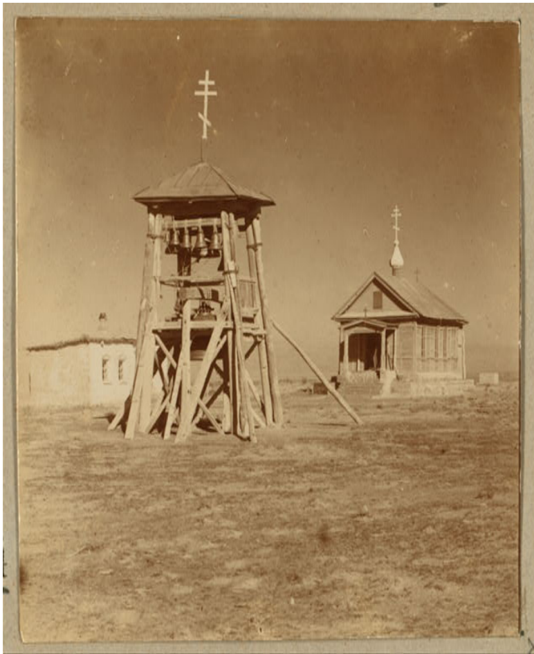
Wooden bell tower, church in Nikolsk settlement, Golodnaia Steppe. 147
